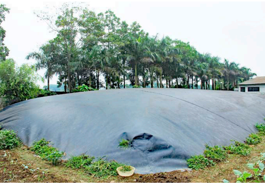
Gastight underground tanks for the production of biogas.
