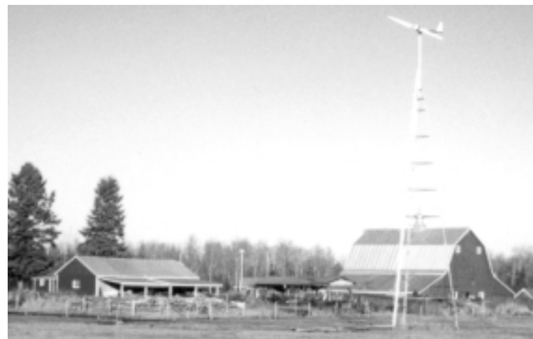
In Clover Valley, Minnesota, this 3-kW Whisper turbine on a 50-foot tower is connected to the utility grid to offset the farm's utility-supplied electricity.
