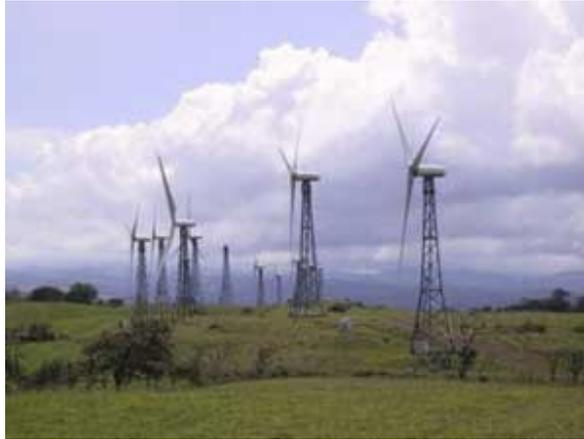
*Wind turbines with steel lattice towers in Costa Rica. ©WWEA e.V.*
